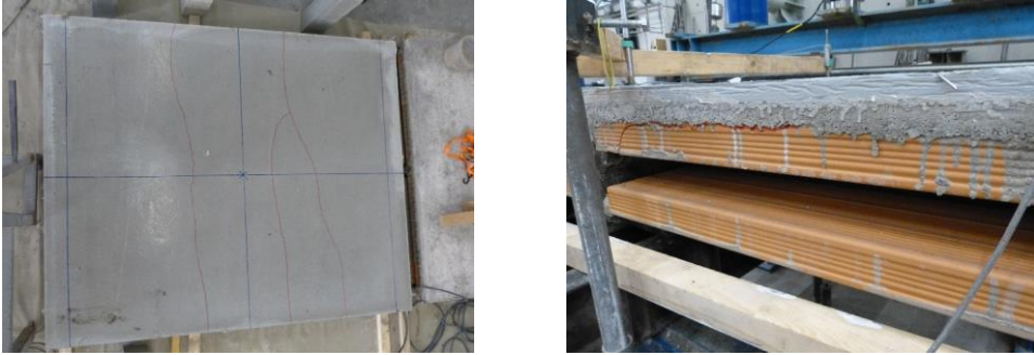
Fig. 7 Condition of the S3 floor before testing: cracking pattern of the slab (left) and tensile failure of the clay tiles.
