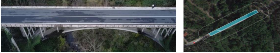
Fig. 2 Bridge subject to inspection (left). Automated flight plan (right)
