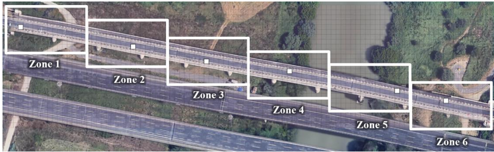
Fig. 5 Bridge's subdivision into zones of interest
