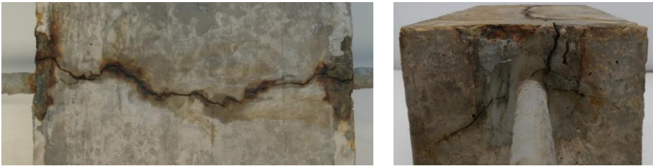
Fig.7 Crack along the specimen.
